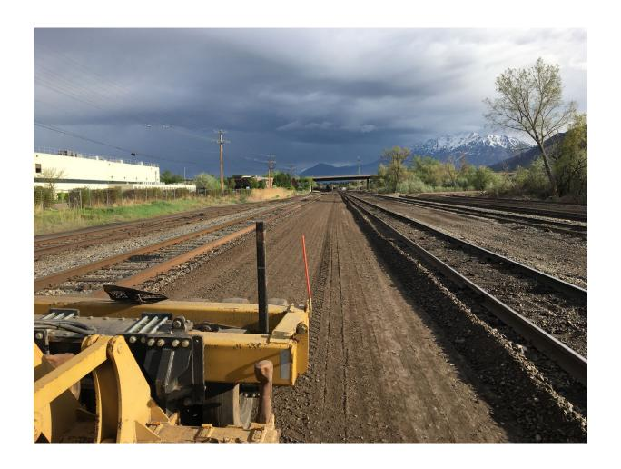
Finish grade prior to Earthbind® Stabilizer topical application. Eliminating the costly aggregate import, by using on site materials.
