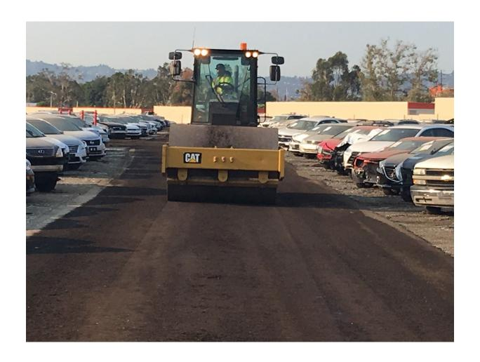
Mechanical rotary mixing of onsite aggregate for a 5" deep stabilization providing long term stability and dust control.
