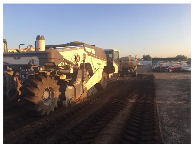
Incorporating on site materials eliminating the aggregate import costs. Mechanical rotary mixing.
